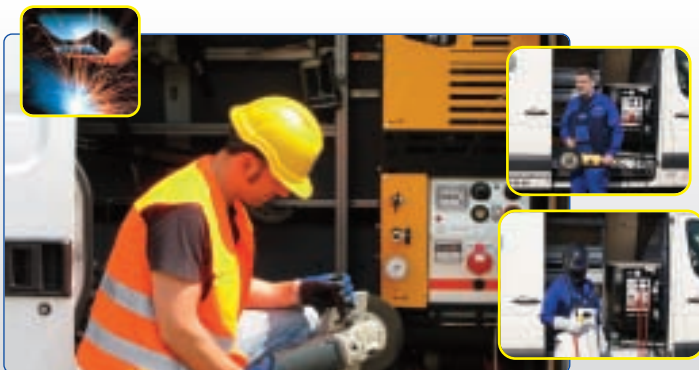
Electricity and welding
